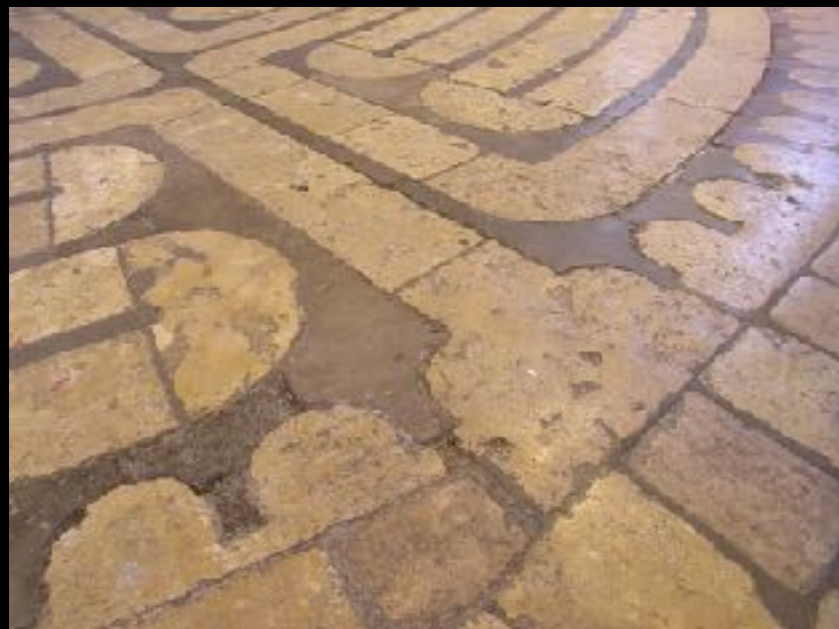
Threshold Stone From the Side
